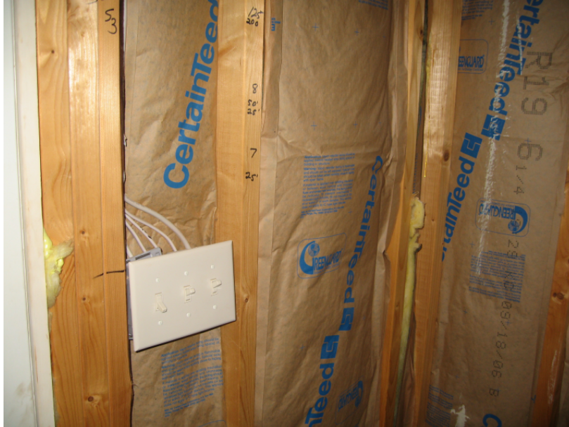
Photo – 6: Inset stapling of the fiberglass allow for convective looping between the kraft paper and the drywall.
